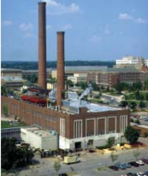
U-M Central Power Plant. Photo courtesy of the University Architect's Office.
